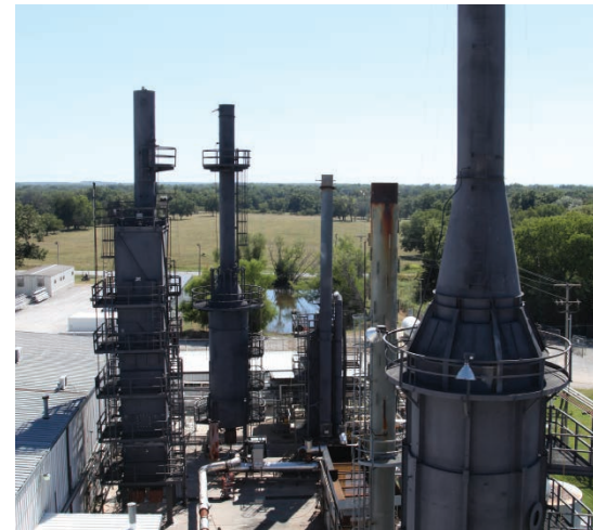
Burner test facility houses seven test furnaces
