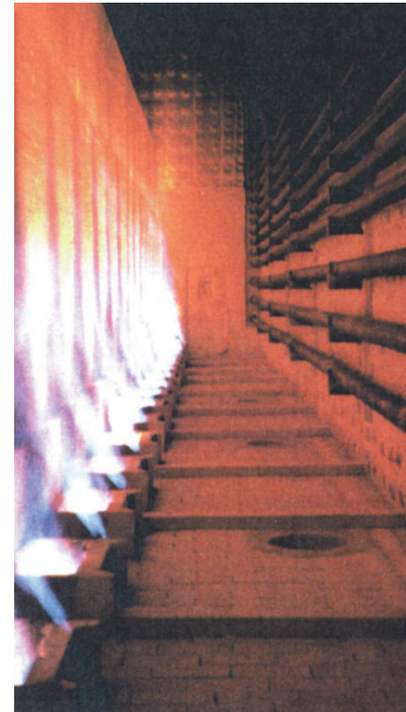
Flat Flame Low NOx Burners
