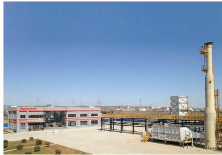
Honeywell UOP Callidus' R&D and Test Center in China
