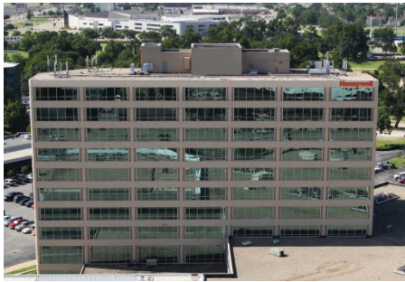
Honeywell UOP Callidus headquarters - Tulsa, Oklahoma. USA
