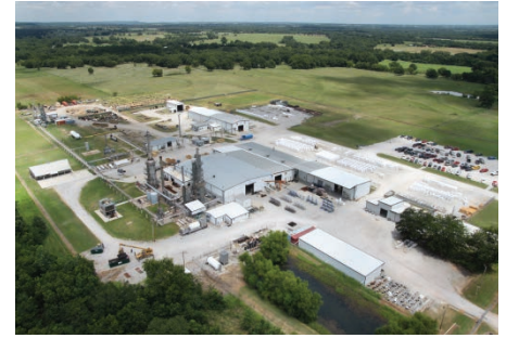
Honeywell UOP Callidus 82,000 sq. ft. manufacturing and fabrication facility in USA
