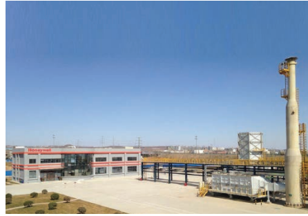
Honeywell UOP Callidus combustion test facility - China
